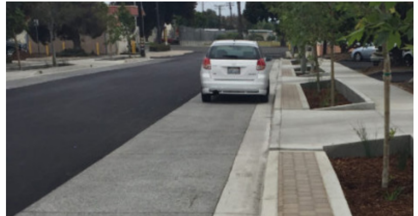
Permeable parking aisles reduce runoff, enhance infiltration
